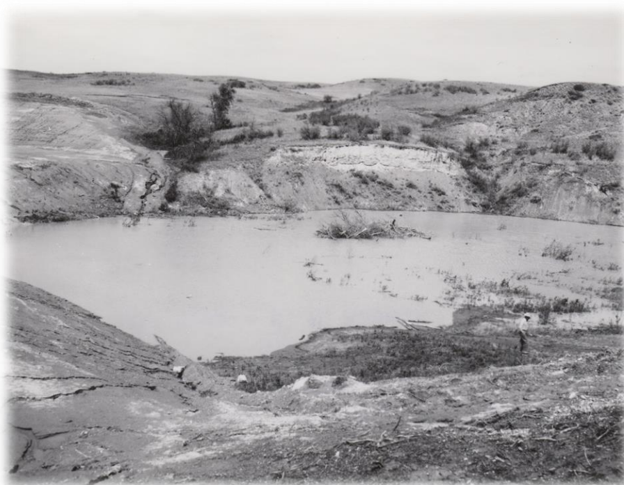
Figure 30. Davis Dam beginning to fill after construction in 1963.
