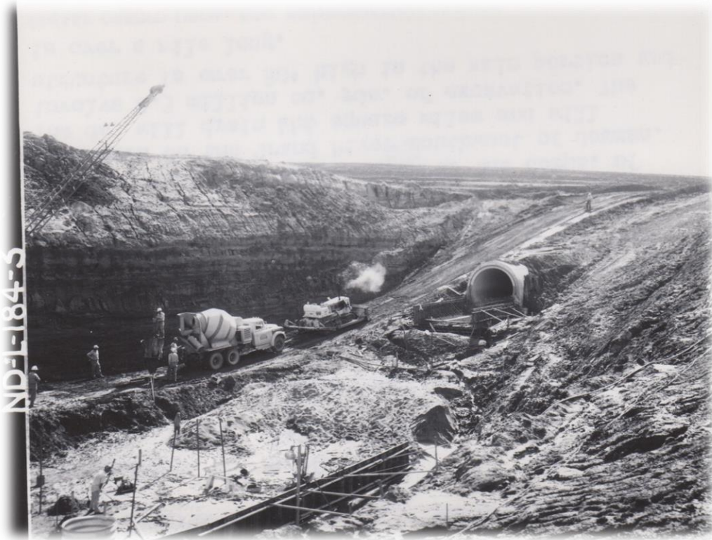
Figure 23. 16-foot concrete principal spillway at the Bowman-Haley Dam. July 1966.
